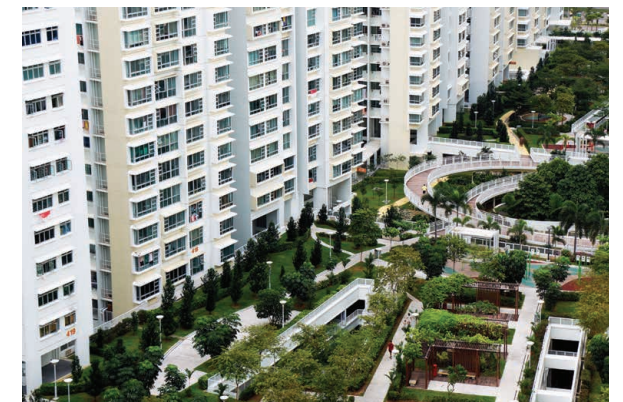
Reducing ambient temperature in housing estates by 4°C through architectural and materials design
