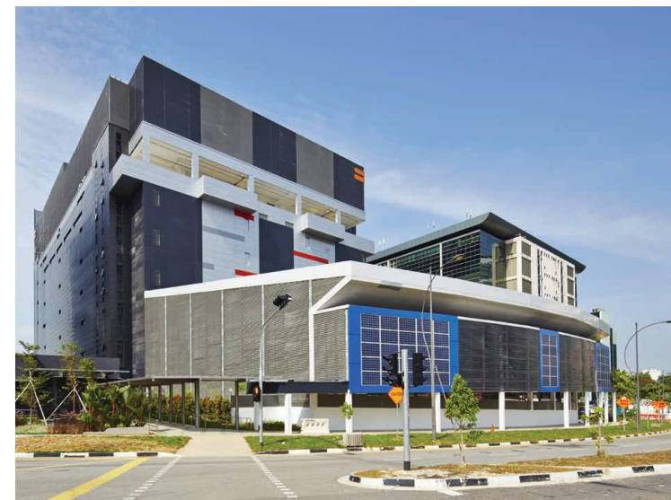
Equinix's Green Mark Platinum SG3 Data Centre in Ayer Rajah Crescent
