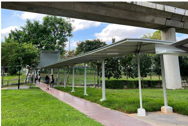
Completed sheltered walkway
